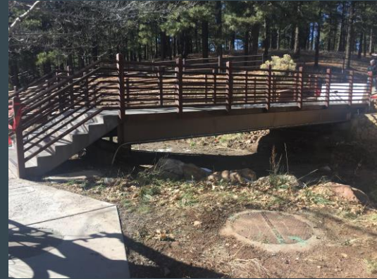
Low Water Crossing at Sinclair Wash [8]
