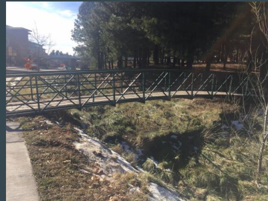
Low Water Crossing at Sinclair Wash [9]
