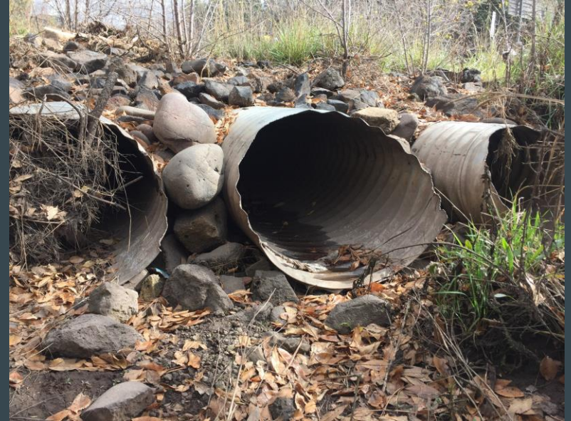
Culverts in Sinclair Wash [4]
